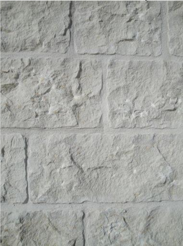
House made of stone blocks "a spacco di cava" (natural split stone)
